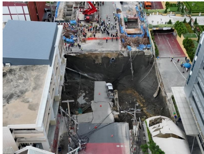
道路の地盤沈下 (出所: Facebook: Office of Disaster Prevention and Mitigation)
